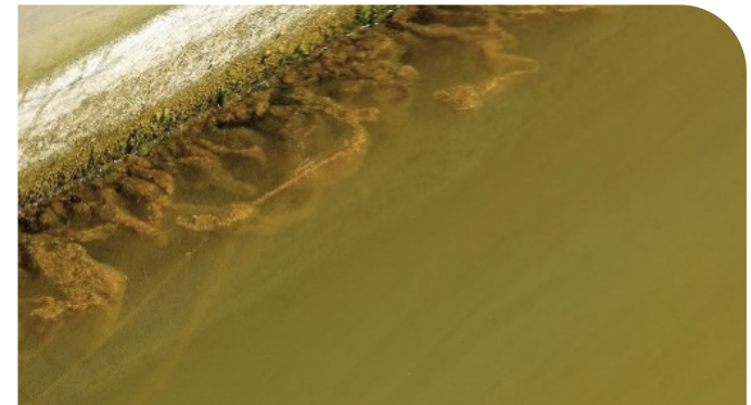
Tower 1: Presence of algae and organic biofilm in the lower part of the tower
