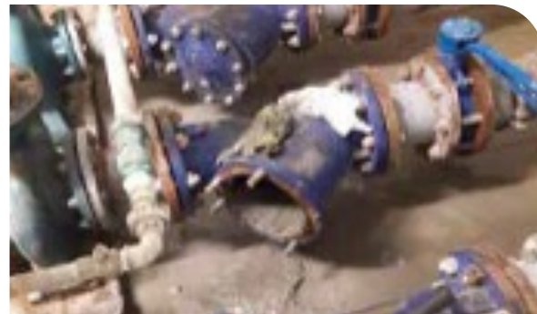
Detachment of encrustations and dissolution of the biofilm
